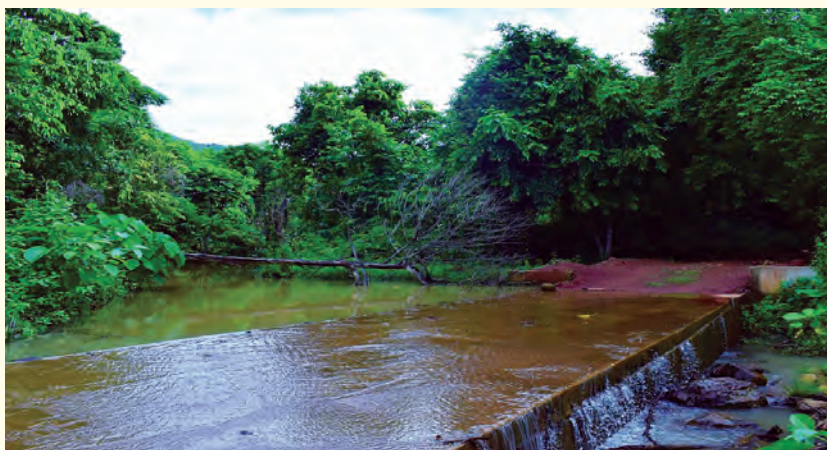
Check dam under Dhenkanal Forest Division
